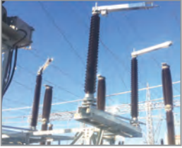
YG KESİCİ - AYIRICILAR (420kV'a kadar) HV CIRCUIT BREAKERS - HV DISCONNECTORS (up to 420kV)
