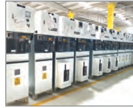
MODÜLER HÜCRELER (12, 24, 36, 40,5kV 25kA'e kadar) MODULAR ENCLOSED SWITCHGEARS (up to 12, 24, 36, 40,5kV 25kA)
