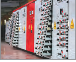
AG PANOLAR (TEDAŞ panolarından form 4b-çekmeceli, 6400A-100kA'e kadar) LV PANELS (from TEDAŞ switchboards type 4b-withdrawable, up to 6400A-100kA)
