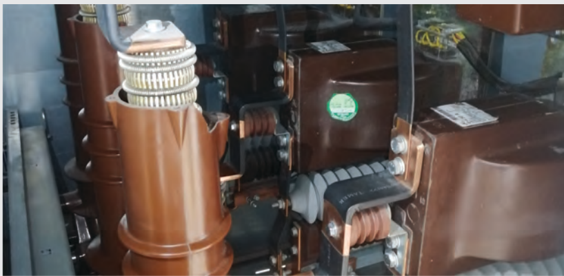
TULIP CLUSTER DRAWER TYPE BREAKER APPLICATION
