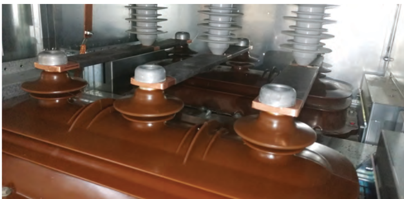
SURGE PROTECTION APPLICATION at MAIN BUSBAR
